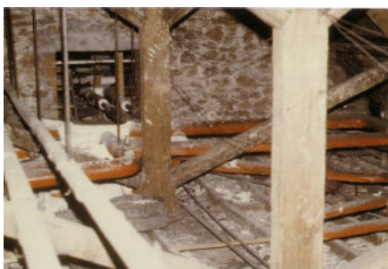
A typical location where asbestos may be found
